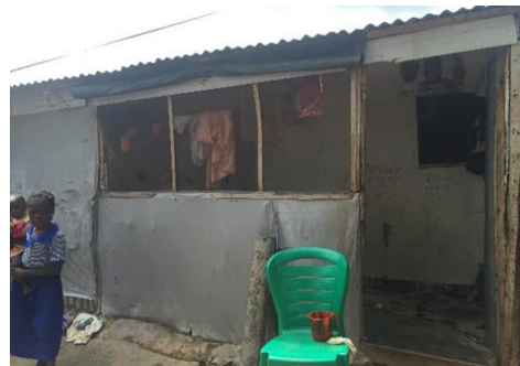
Figure 8: Karmajiji camp Accommodation, built as a permanent structure. Picture taken in 2016
