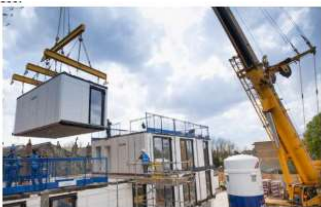
Figure 2.1: Installation of Modular Home
