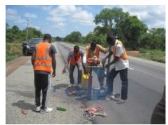
Fig. 2. Coring through the pavement structure..
