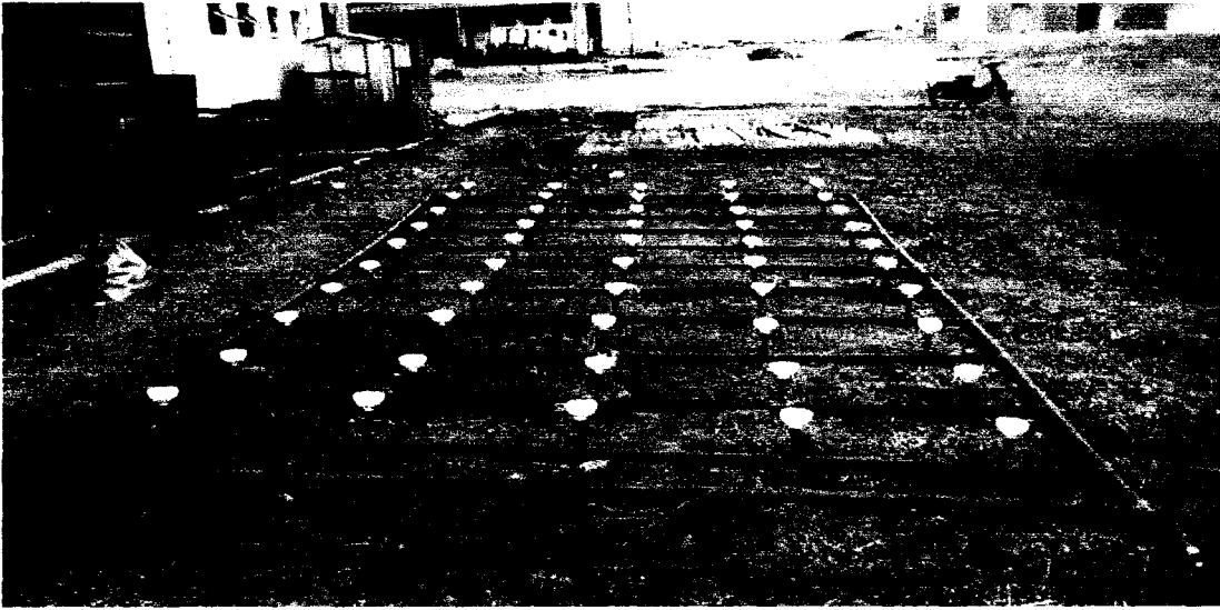
Plate 1: Construction of Rainfall Simulator
