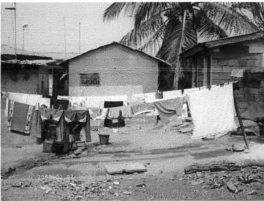
Plate xi Resettlers' House with structural modification In Kubwa Resettlement Town
