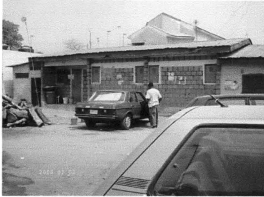
Plate x Resettlers' House devoid of structural modification In Kubwa Resettlement Town
