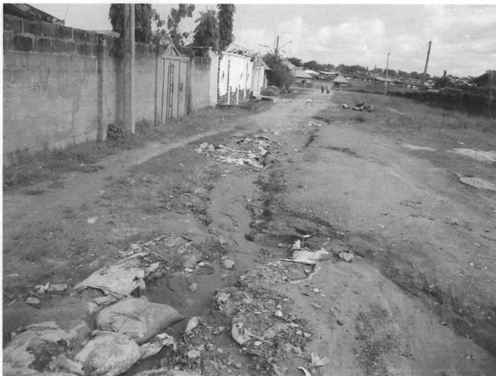
Plate X. Erosion Caused by the Removal of Natural Vegetation, Bosso Estate.
