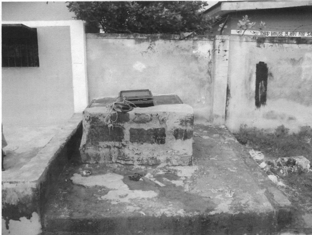
Plate VII Hand Dug Well used as a Groundwater Source.
