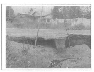
Plate xiii Shoulder failurePlate ix Base Shears within Sub - GradeSource: Author's field work, Zuba -Gwagwalada, 2007
