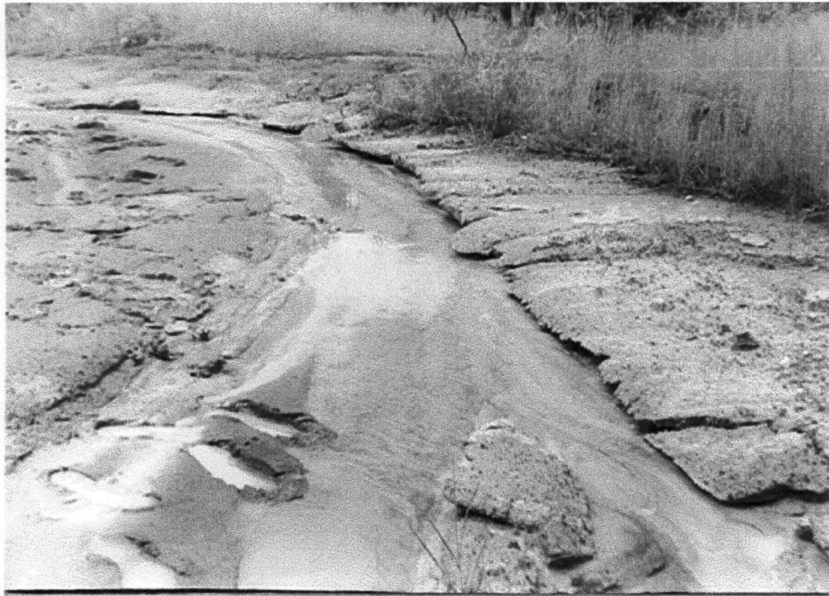
Development of gullies on tract/road network within the Park.
