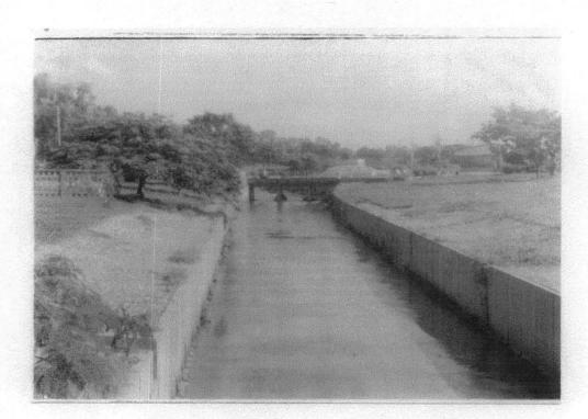
Plate 1: The drainage channel that cut across the Bosso camus of F.U.T, Minna, Was concretized to protect the Bank against collapsing.
