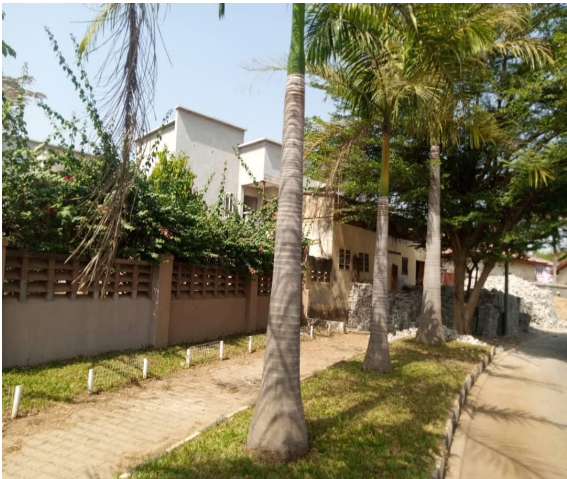
Plate III: Image of Building Affected by Obsolescence and Adjoining another residential building in Wuse Abuja.
