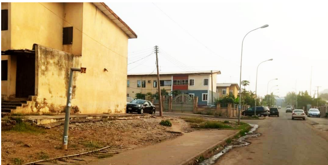
Plate II: Image of Building Affected by Obsolescence and Adjoining Properties in Garki Abuja.
