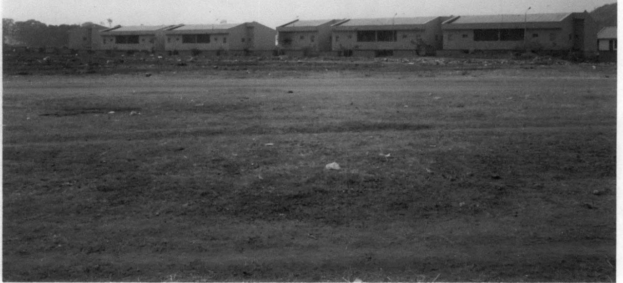
PLATE 1: Area behind National assembly quarters, Garki II.
