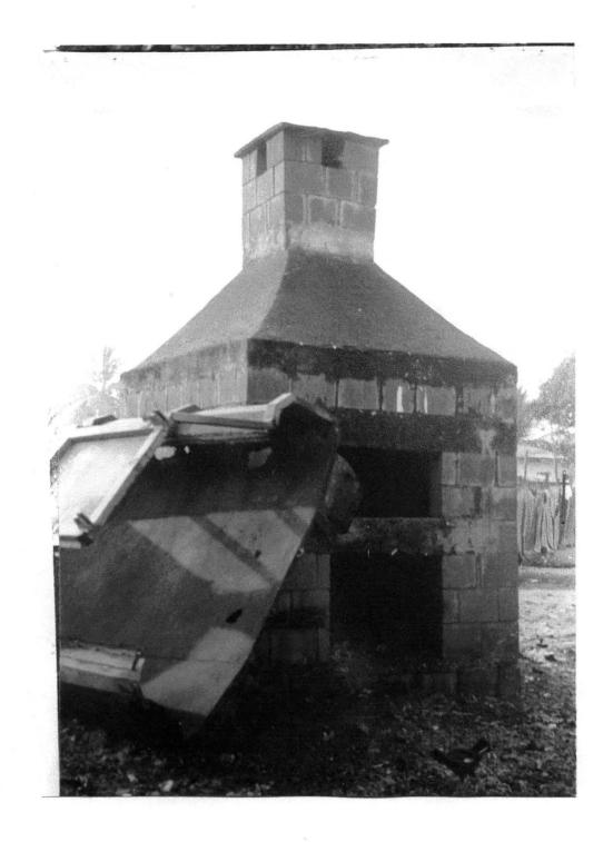
**PLATE 3.** An incinerator where controlled burning of combustible solid wastes takes place.
