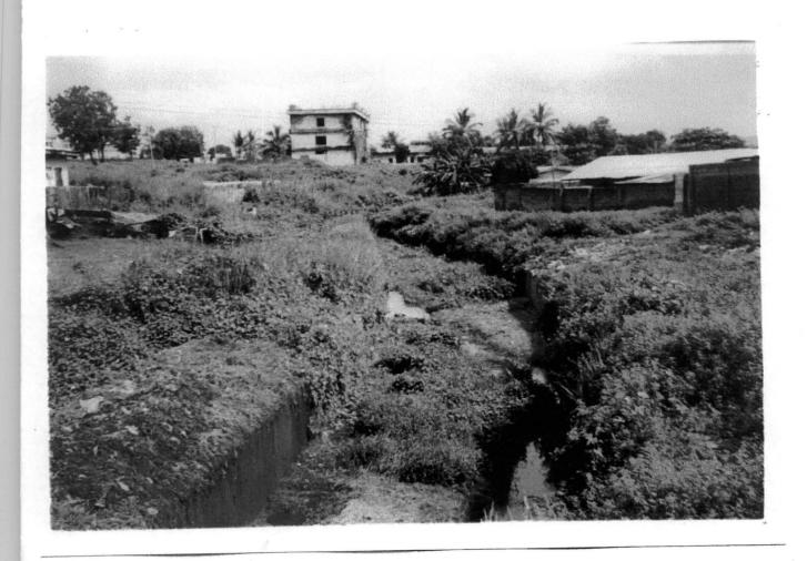
**PLATE 4.** A section of modern drainage system in Minna. Note the presence of refuse on both sides of the embankment. The refuse is also seen falling into the drainage. Also to be noted is the accumulation of wastes and the growth of weeds inside the drainage fertilized by the falling wastes.
