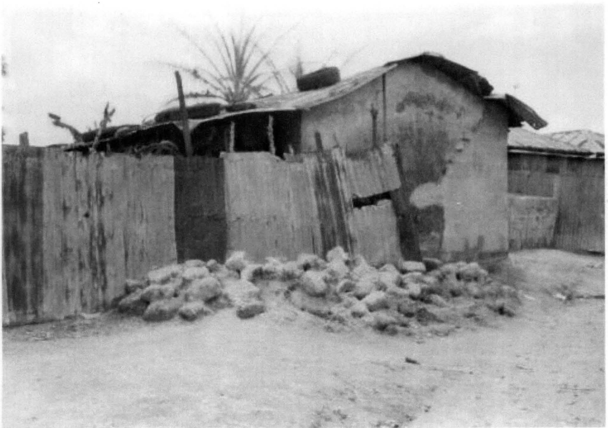
Plate II: Showing building partially collapsed (although re-built)
