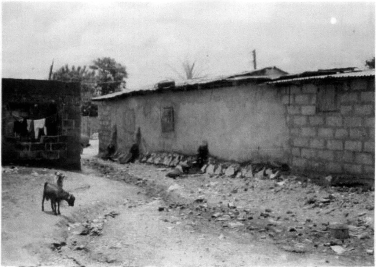
Plate VII: Showing a collapsed (but re-built) building
