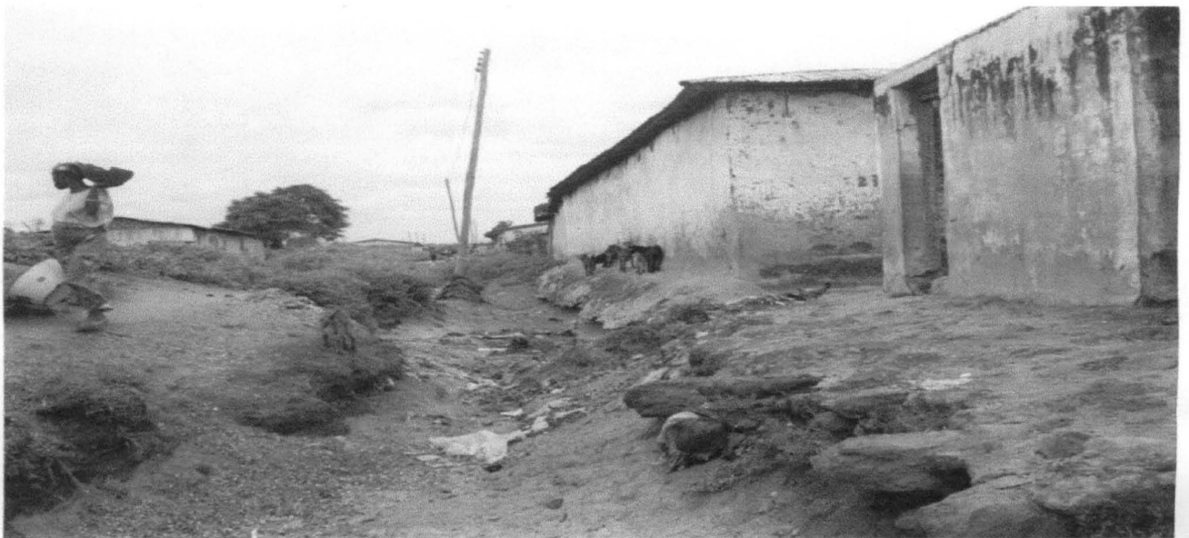
PLATE 5.12 to 5.14: Shows houses under great threat due to erosion activities in Army Barracks SOURCE: Field Survey, 2001
