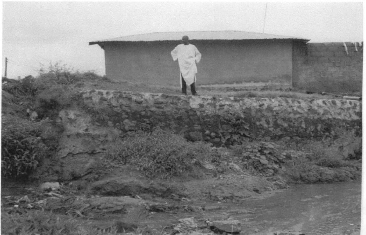
PLATE 5.16: Shows traditional stone pitching work to present erosion
