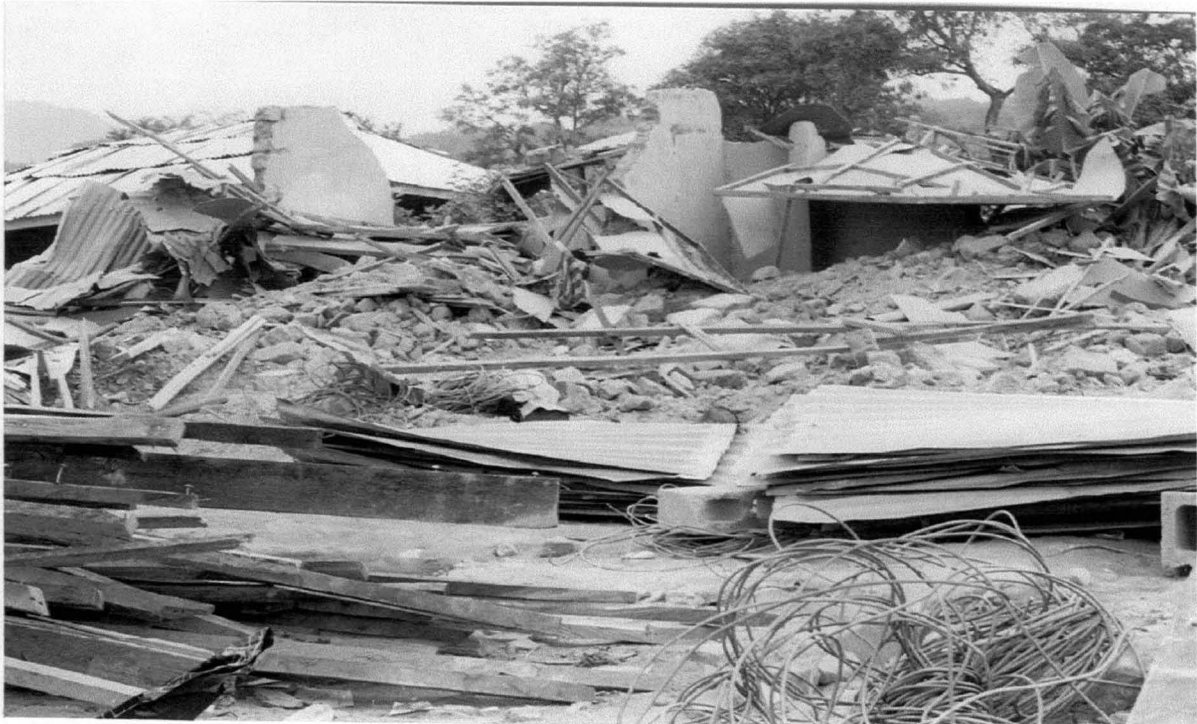
Plate 4. 4 Demolition in Karimajiji
