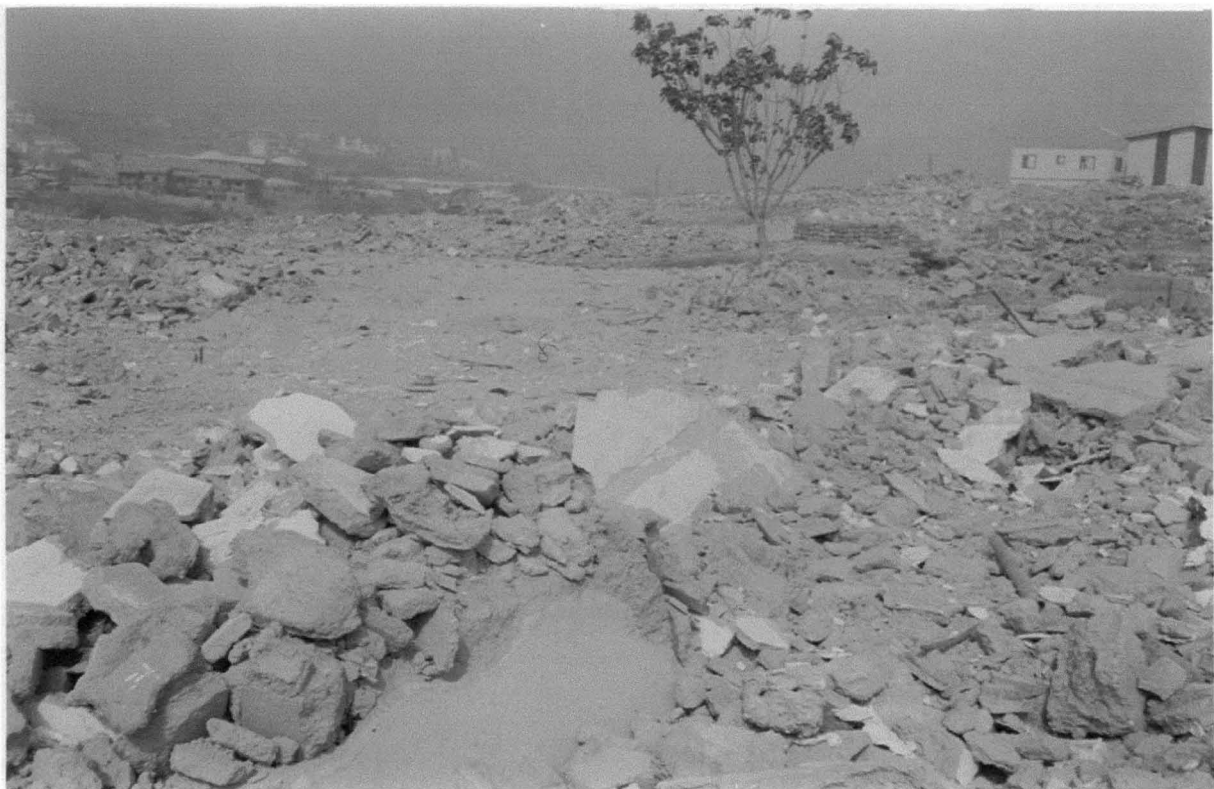
Plate 4. 2 Demolition in Nyanya
