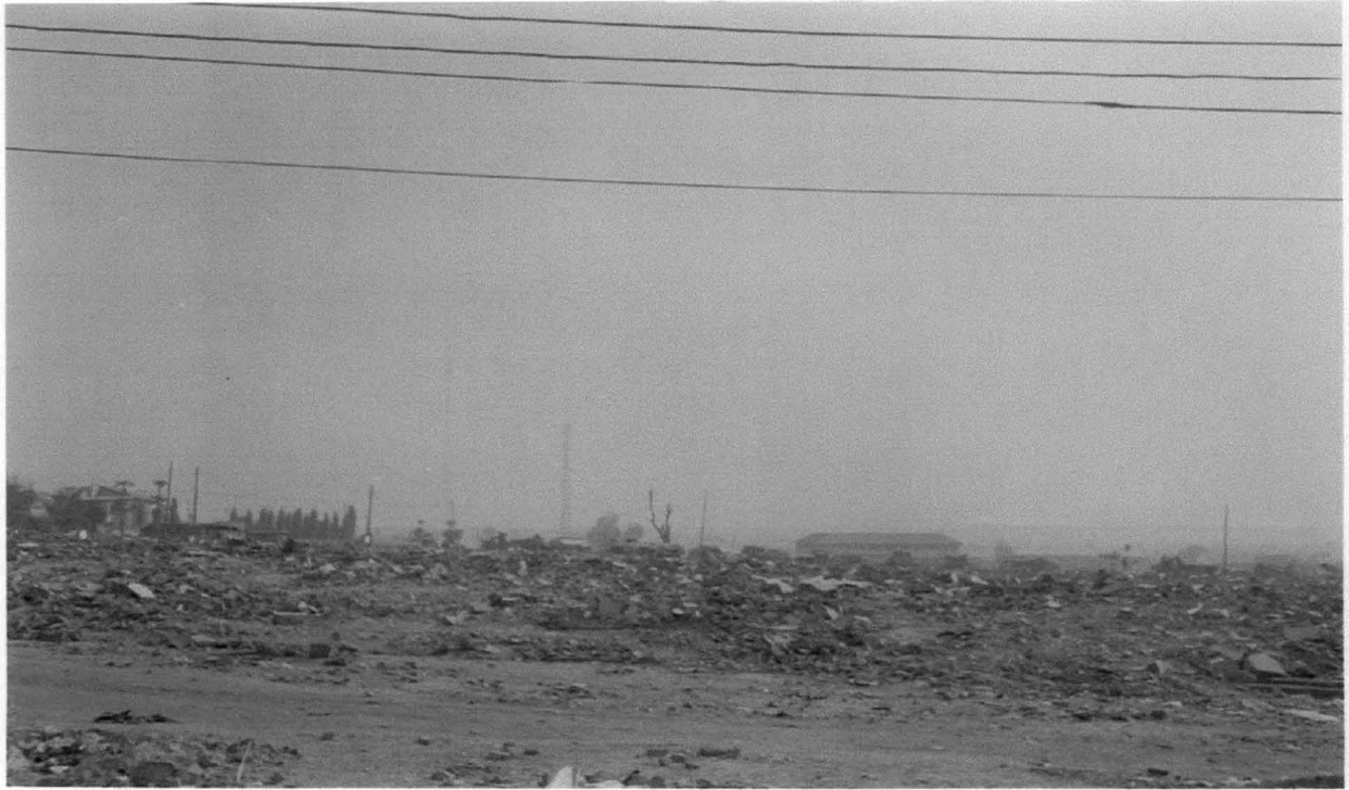
Plate 4. 3 Demolition of Tipper Garage, Nyanya
