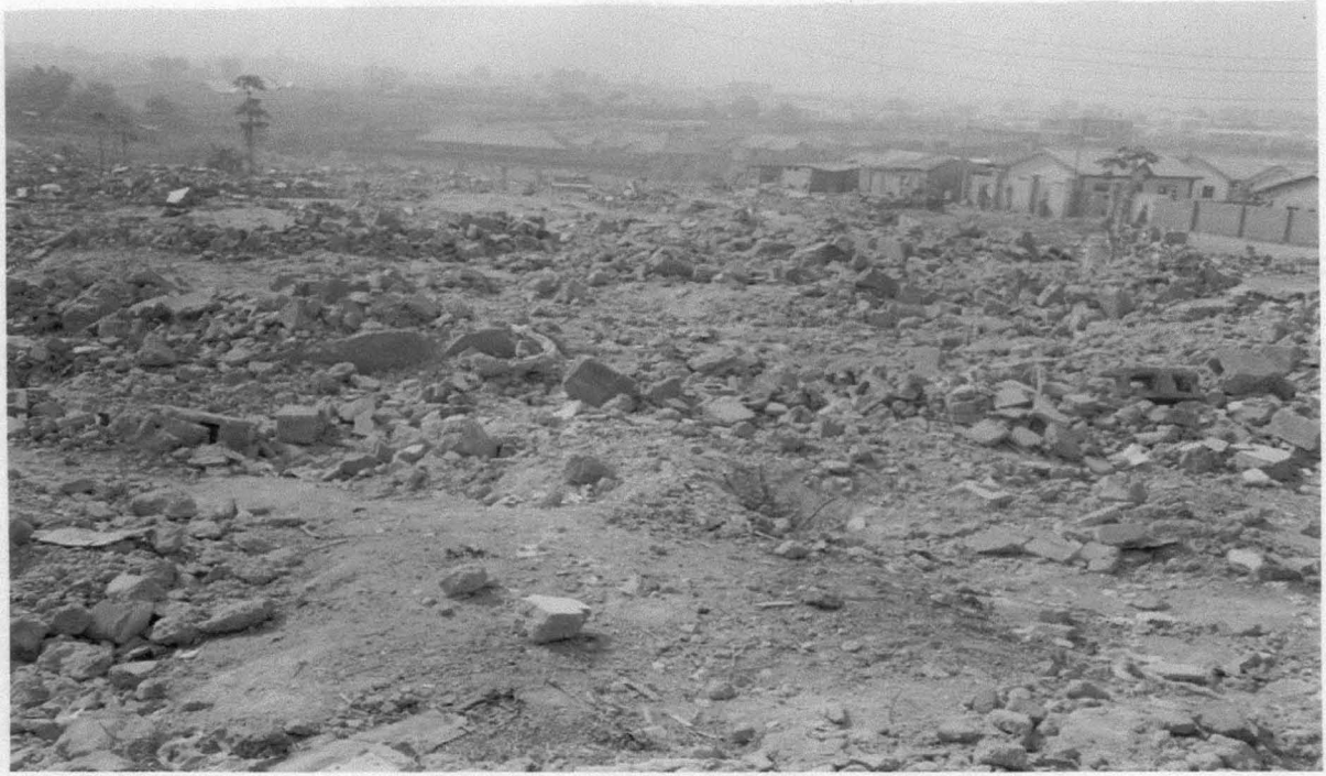
Plate 4. 1 Demolition in Karu
