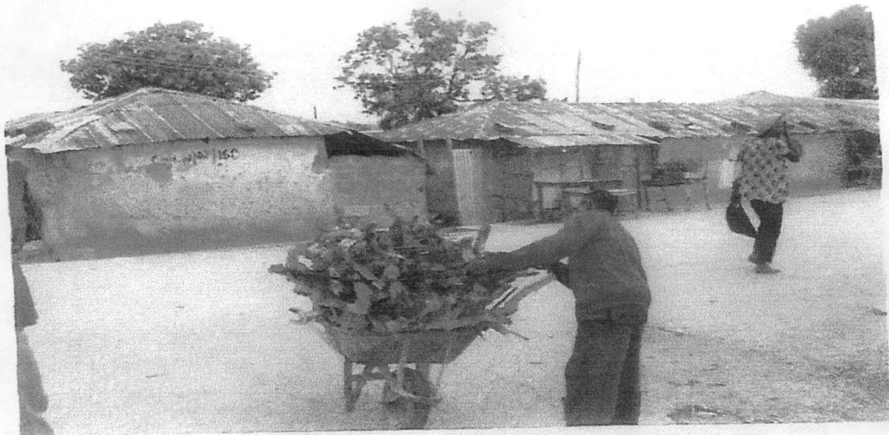
Plate 7: Shows large stone and block placed on roof top to prevent roofing sheet from been blown off by wind. Also shown the effect of rain on wall discolouring and flaking the rendered wall
