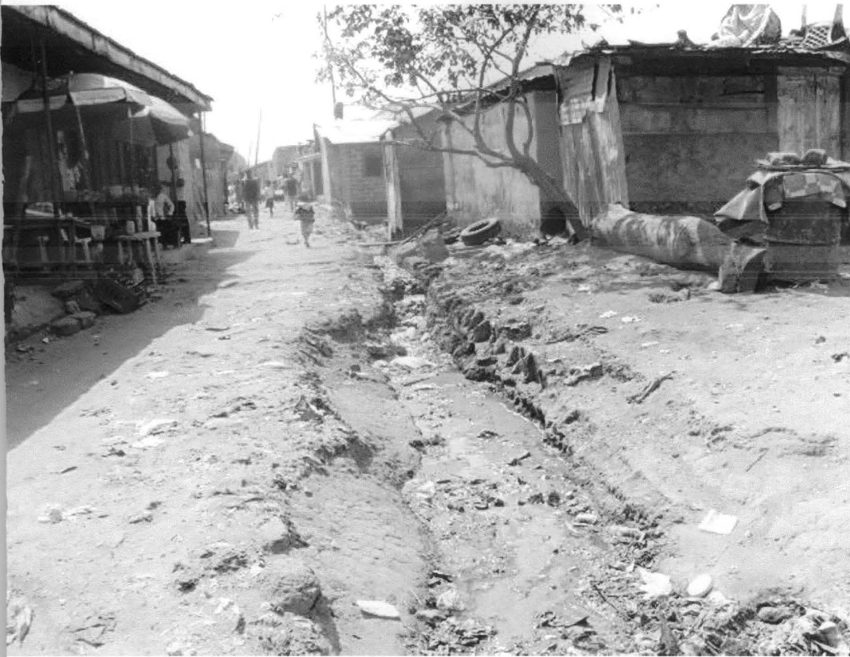
PLATE III: POOR DRAINAGE SYSTEM (SITE B)
