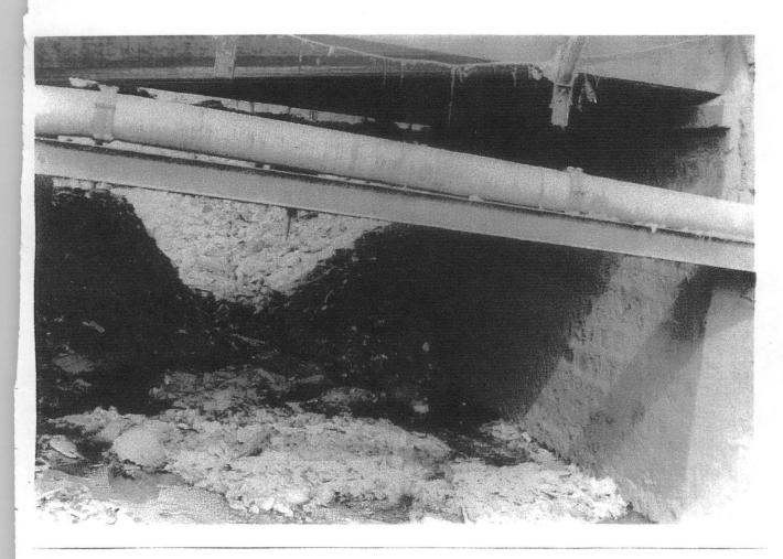
Plate 7: Refuse blocking a concrete Bridge in Suleja.
