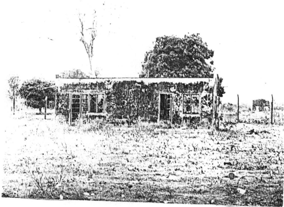
Plate 3. Defects in roof
