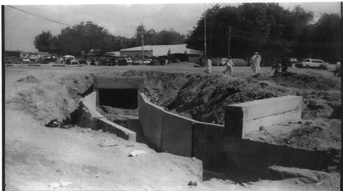
Plate 6: Construction of drainages to discharge water from Rafin Atiku pond
