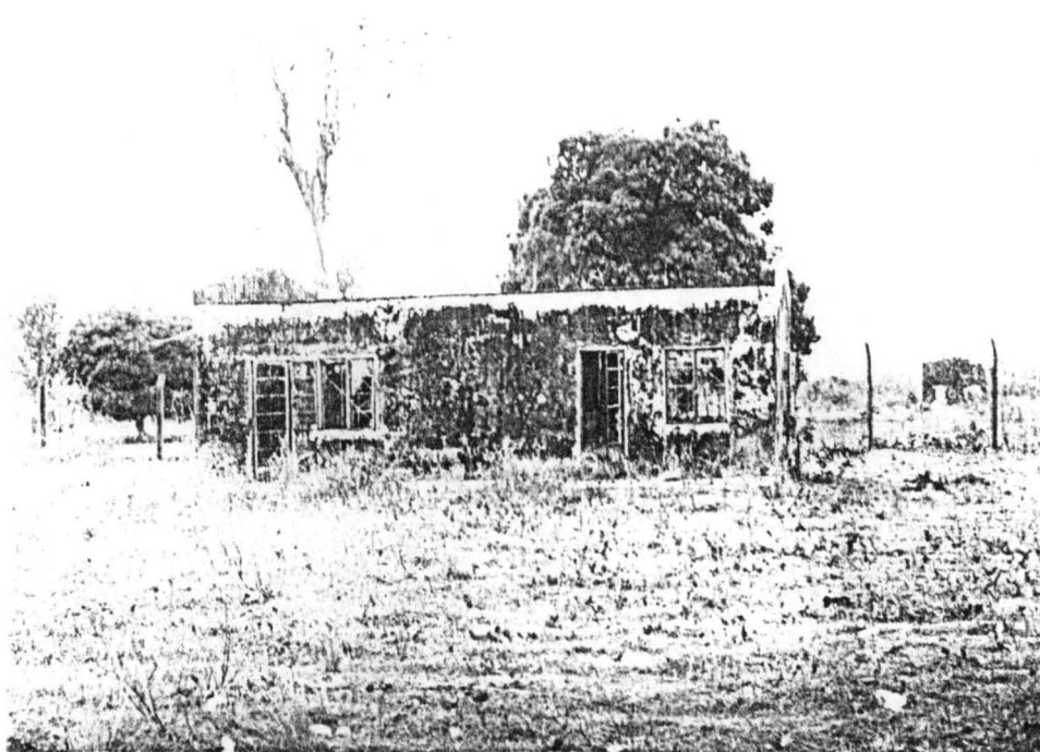
Plate 3. Defects in roof
