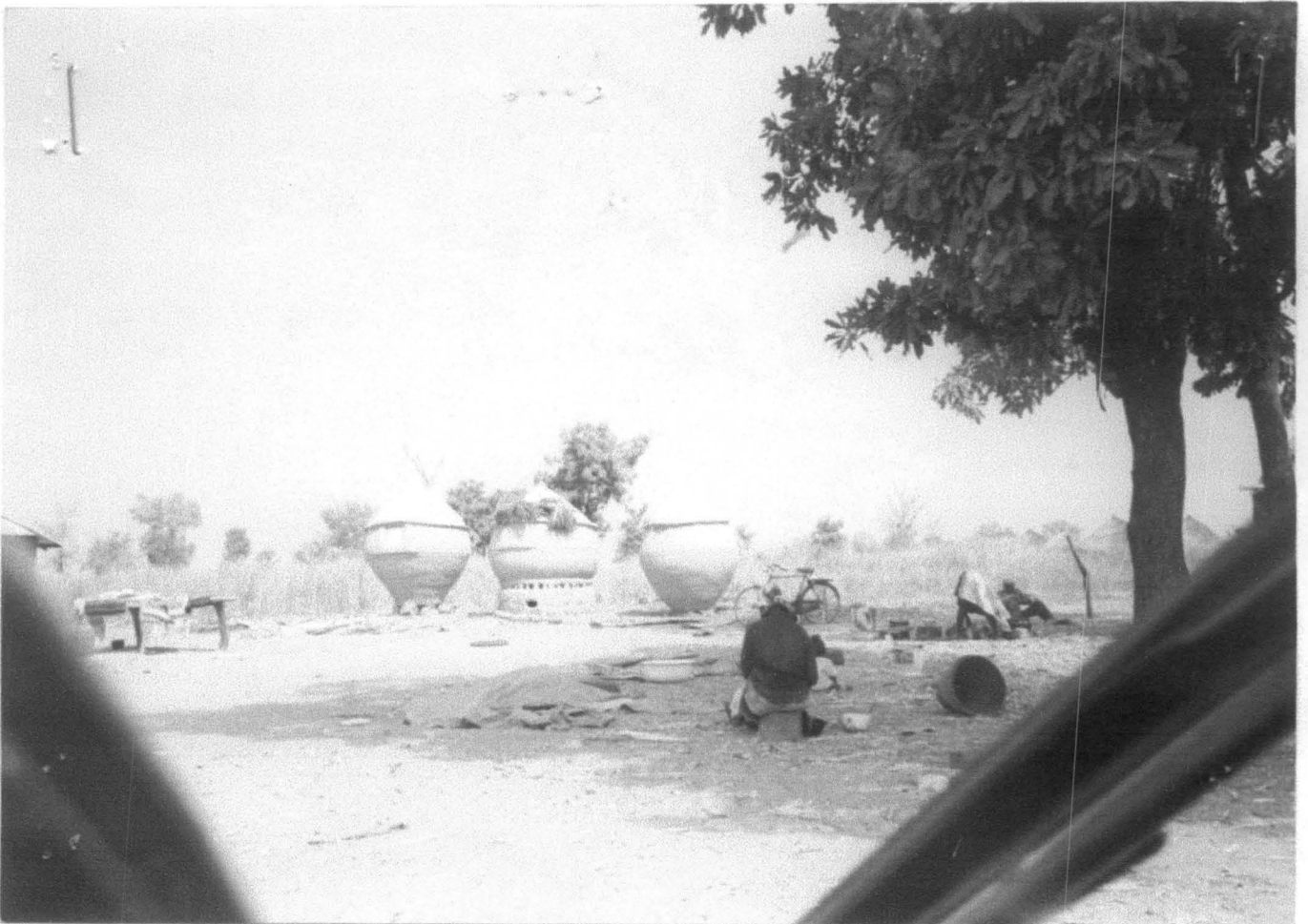
Local grain storage structure at Yabatagi in Niger State.
