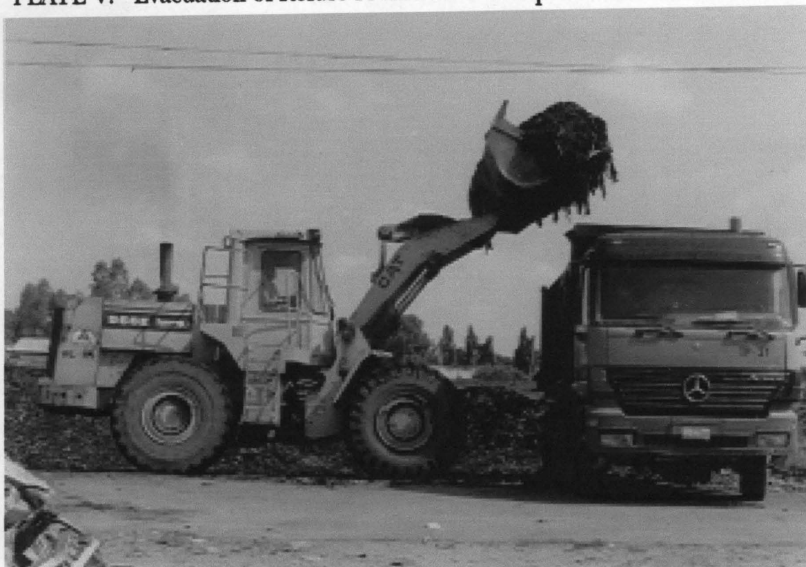
Source: Field Survey October, 2004
