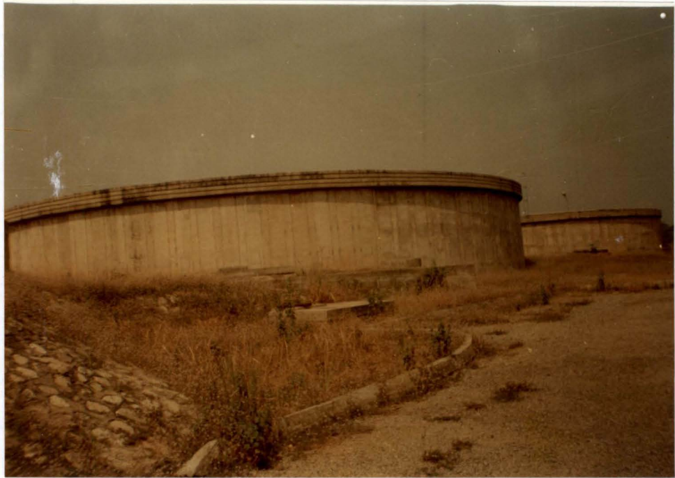
BALANCE/CLEAR WATER TANKS. EACH TANK HAS THE CAPACITY OF 4300M**3.
