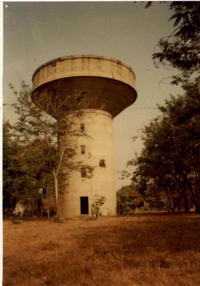
G.R.A. ELEVATED RESERVOIR. CAPACITY 900M**3
