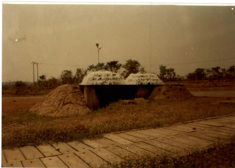
AERATOR, THE RAW WATER OUTLET
