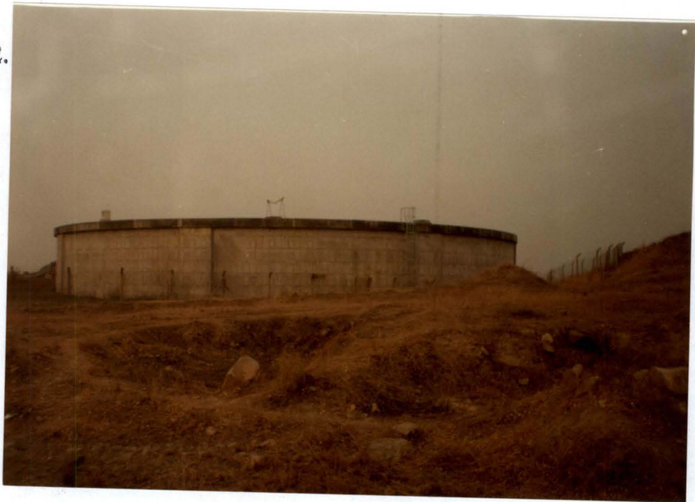
NEW MALONEY HILL SERVICE RESERVOIR. CAPACITY 12'500M**3
