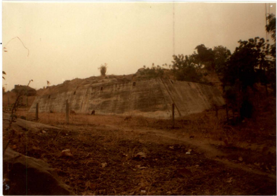
OLD MALONEY HILL SERVICE RESERVOIR (GROUND CEMENT) CAPACITY 1000M**3.
