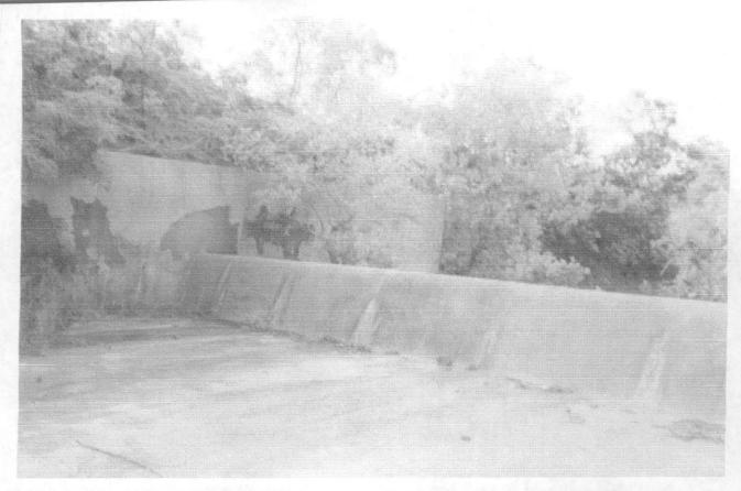
Plate 12:- Showing Eroded fringes of the reservoir at the Spillway.
