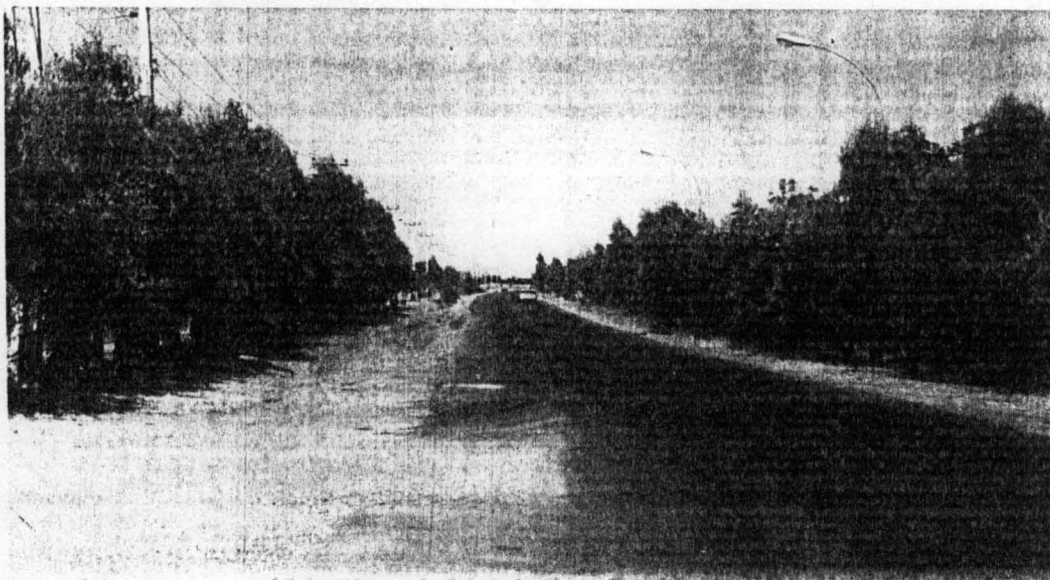
Plate 4.1b Windbreak Plantation for Desertification Control SOURCE: Field Survey
