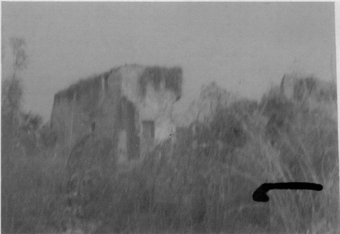
Plate 12: showing Monumental Upstairs in Bosso Village (Dilapidated)
