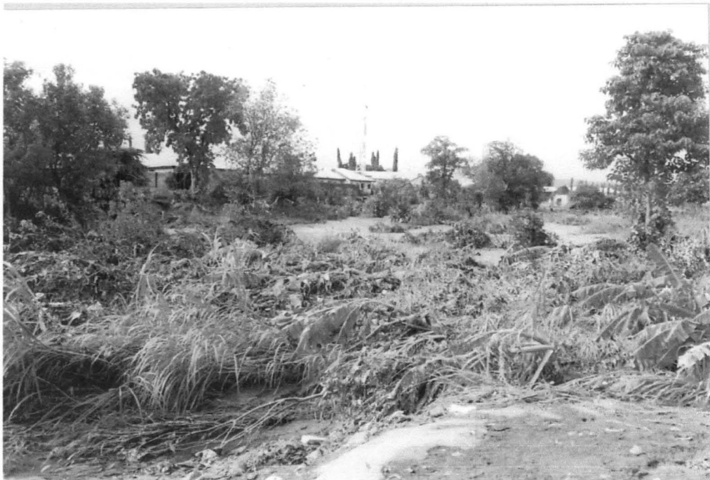
Plate II: Ravaging effect of flood in F.H.A. estate phase III Kubwa
