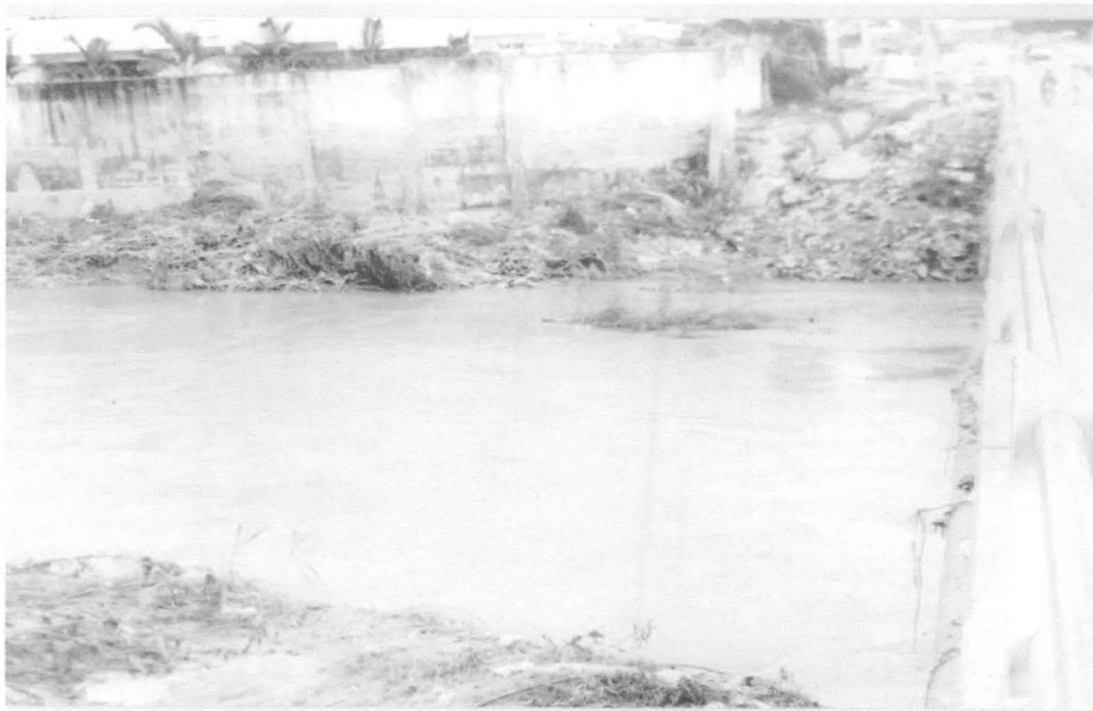
Plate VIII: Indiscriminate dumping of refuse in the phase III Kubwa river by the adjoining buildings in the flood plain
