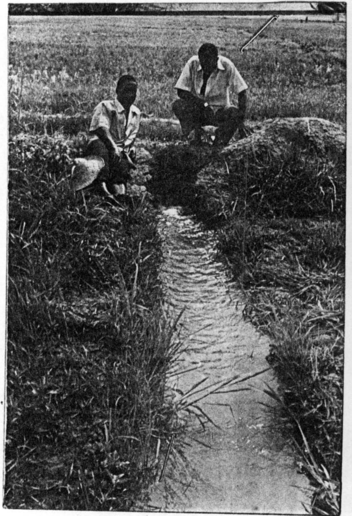
Fig. 7b. Downstream view of the Pipe Outlet.
