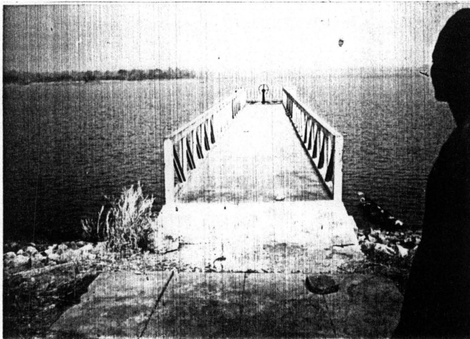
Fig. 3: Upstream view of Tunga Kawo Dam with slide gate.
