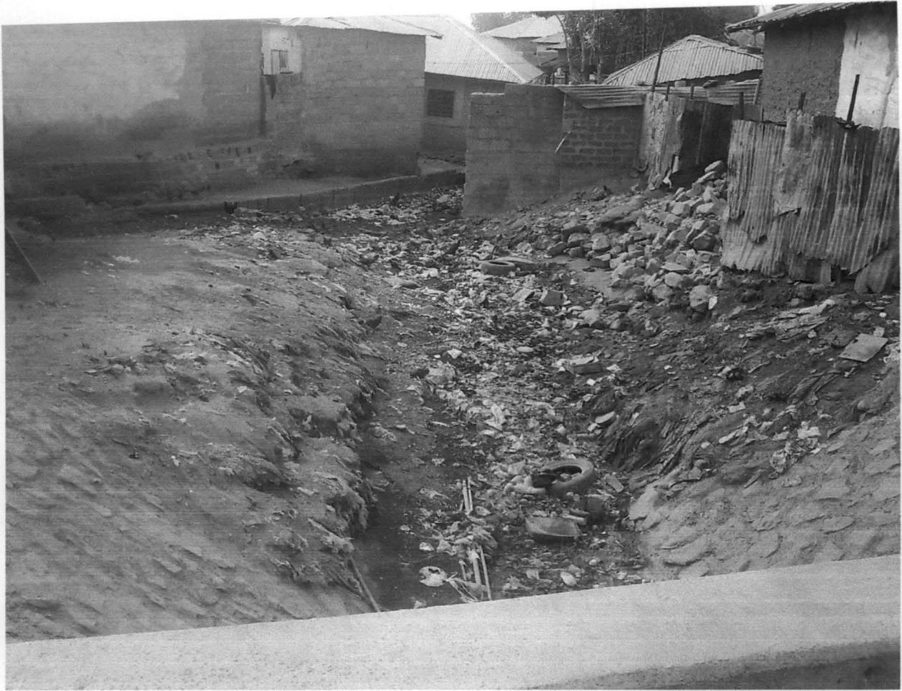
Plate I: Drainage Littered with refuse at Karofi; An area classified as High density
