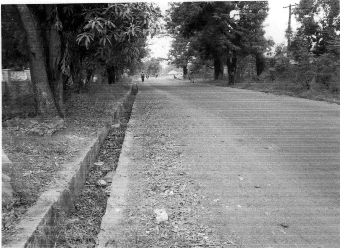
Plate V: Drainage littered with dry leaves at GRA; An area classified as Low density
