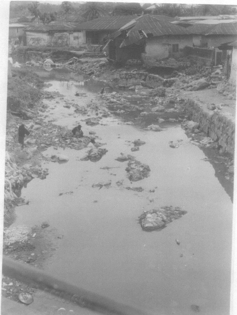
4.1g: Dawaki Junction – Kantoma – Channel uncovered by Township Erosion Control Project. Showing Diverstating effect on building and other structures.
