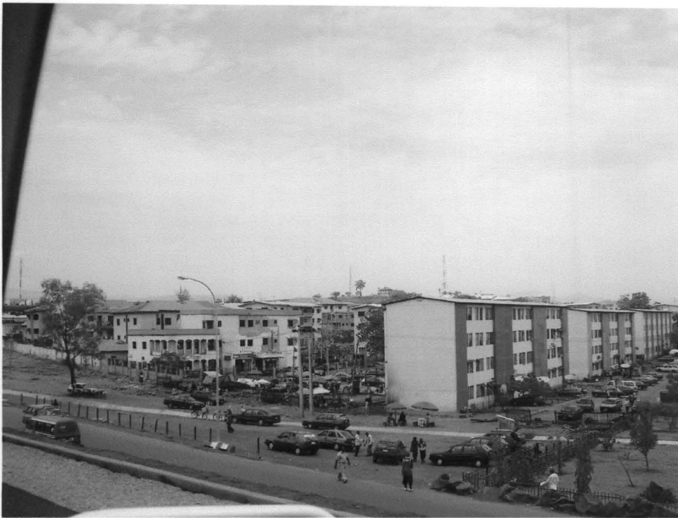
Plate V: The residential building within the study area that replaces vegetation.
