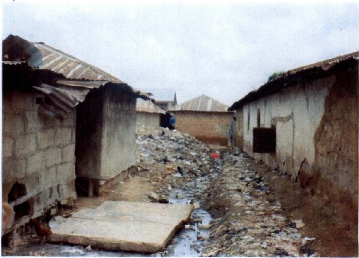
Plate V: Showing bad drainage and poor waste disposal system prevalent in the study area
