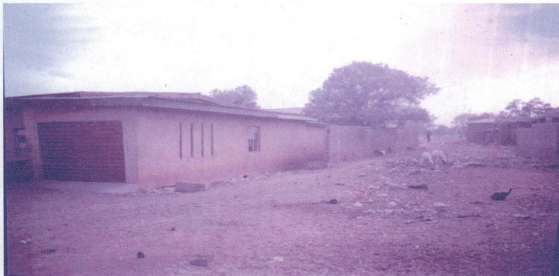
PLATE I SHOWING FALLEN FENCE EMIN-NDAGBODO
