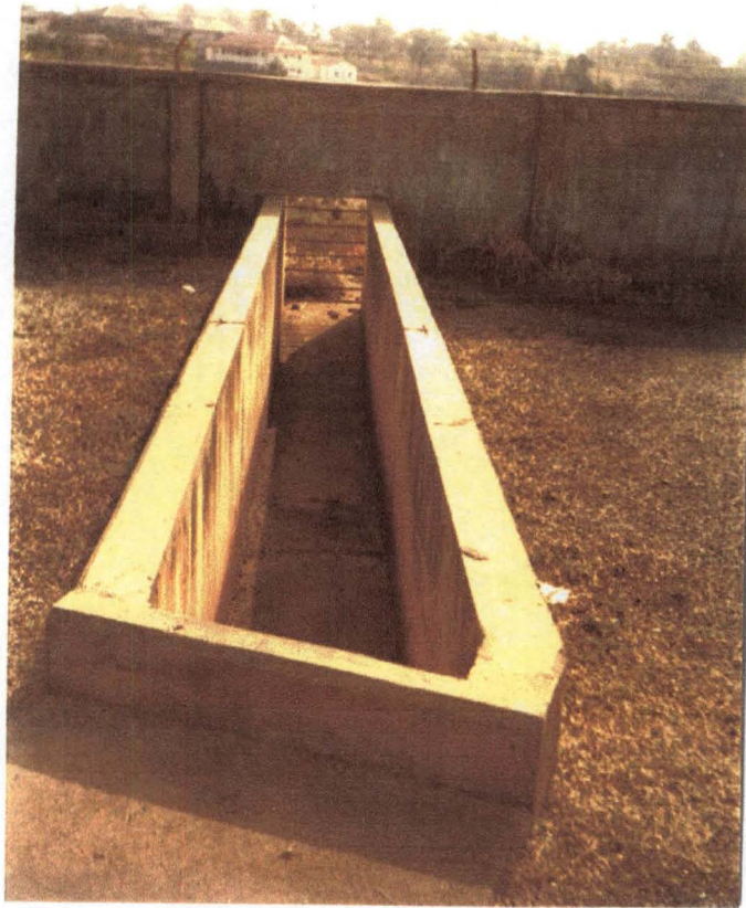
PHOTOGRAPH 1X Outlet of Treated Sewage into Wuye River
