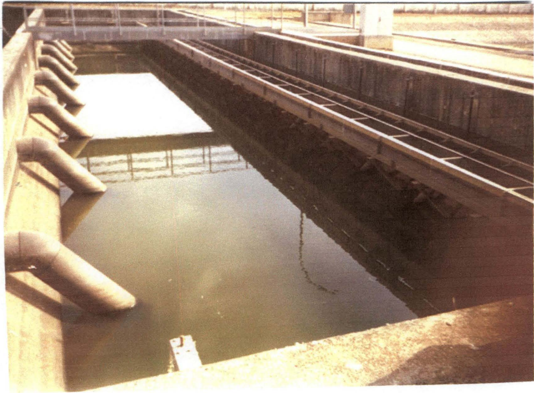
PHOTOGRAPH V Sewage from the Aerator to the various ponds
