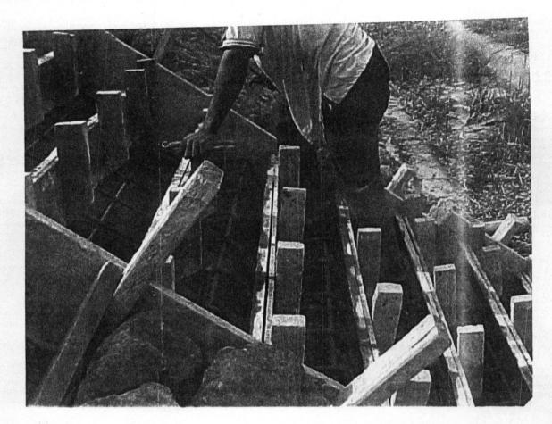
**GROUP O :** MISCELLANEOUS PROTECTION WORK; FORMWORK AND REINFORCEMENT FOR STAIRCASES AT THE UPSTREAM SLOPE OF THE ACCESS ROAD BESIDE OLD RELIEF WELL AND MAIN DAM ENCAPSULATION BERM.
