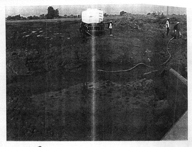
GROUP &: MAIN DRAINAGE CANAL NO.1, PLACEMENT OF FILTER BEDDING.
