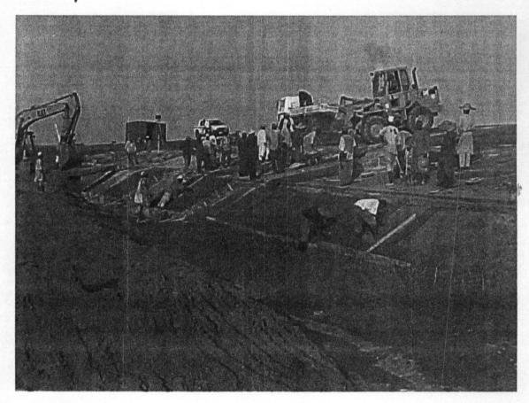
GROUP HA: EMERGENCY SPILLWAY; BLINDING AND CASTING OF SLAB.
