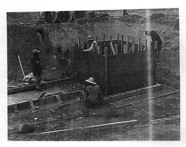
**GROUP A:** MISCELLANEOUS PROTECTION WORK: KETA 900mm DIAMETER RING PIPE CULVERT ; BLINDING, REINFORCEMENT AND FORMWORK FOR THE SUMP.
