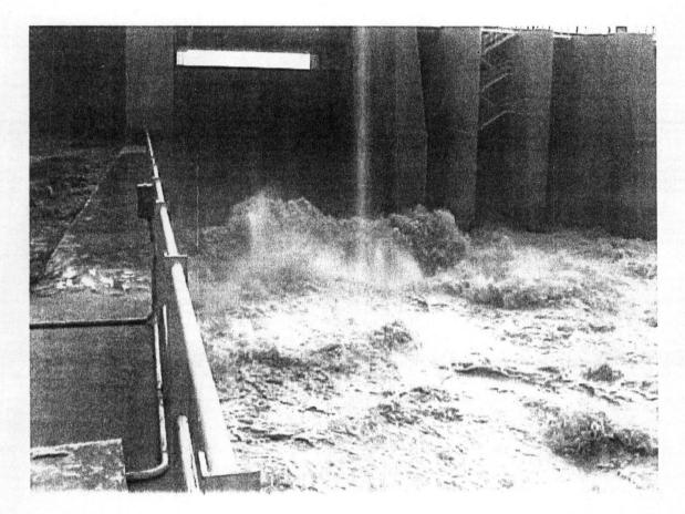
GROUP HA:SPILLWAY GATES FLOOD DISCHARGE : MONTH OF SEPTEMBER WITNESSED A PEAK DISCHARGE RATE OF 400m<sup>3</sup>/s
