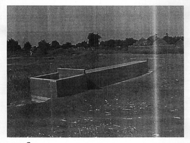
GROUP S: MISCELLANEOUS PROTECTION WORK: COMPLETION OF 1990 900mm DIAMETER RING PIPE CULVERT. 69
