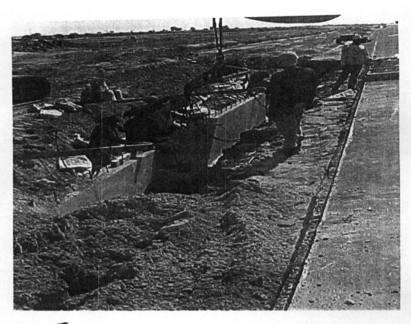
GROUP 12 : EMERGENCY SPILLWAY; PLACEMENT OF ANCHOR BEAM.
