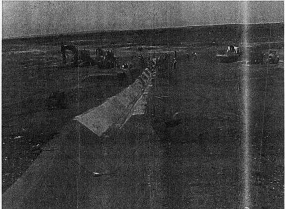
GROUP A: ROAD SECONDARY- SADDLE DAM ; CONCRETE LINED DRAINAGE CHANNEL TOWARDS INLET OF CULVERT AT CH 0+090.
