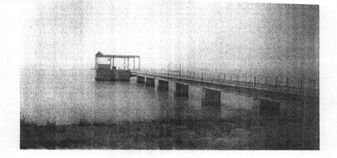
ATE NO 9: ACCESS BRIDGE LEADING TO THE BULKHEAD GATE CONTROLLING CRANE AND METEOROLOGICAL EQUIPMENT.
