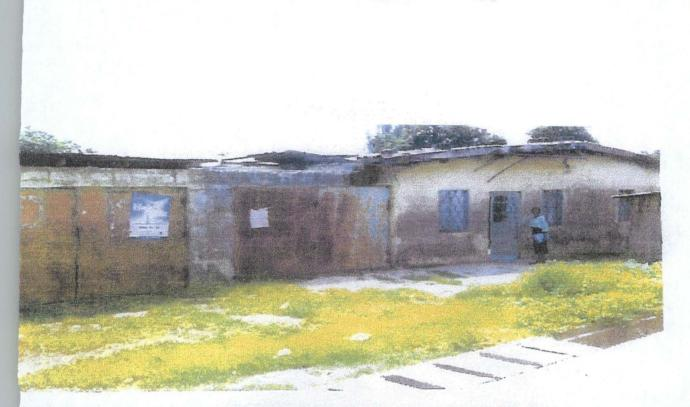
Plate 1: The effect of rainstorm on a house; Wind has blown off Part of the roof, discoloured paint surface, corroded metal gate, roofing timber, fasica, board and ceiling board decayed due to moisture.
