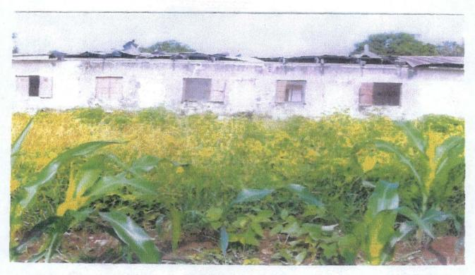
Plate 6: The effect of rain washing away the paint on wall and Wind blowing off part of the roofing sheet. Also part of Fascia board and ceiling board completely falling off in G.T.C. Minna. Source: Field Survey
