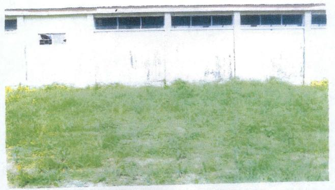
Plate 11: Shows the effect of rain on wall surface washing off the paint on a workshop block in G.T.C. Minna in Chanchaga town.
