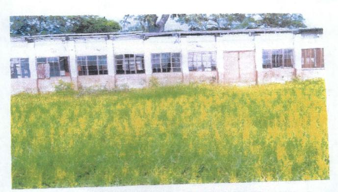
Plate 5: Shows the effect of wind blowing off roofing sheet of classroom block in Government Technical College Minna in Chanchaga town.
