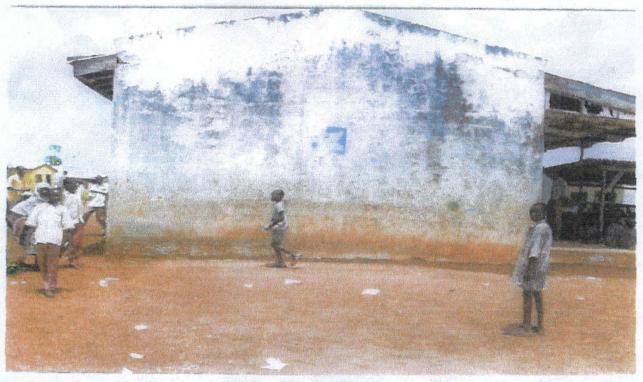
Plate 12: Shows the wall of a Primary School in Chanchaga with washed off paint surface, flaked rendered wall and damped fascia board with decayed ceiling board.
