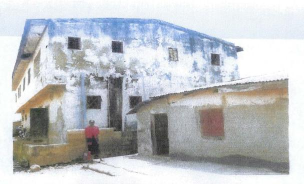
Plate 9: Shows the effect of rain on a storey building washing of the paint and damp penetration at the top part of wall surface.
