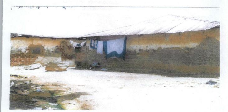
Plate 4: Shows the effect of rain which have wash off the paint and peel of the rendering exposing the mud and sandcrete block in Chanchaga town.
