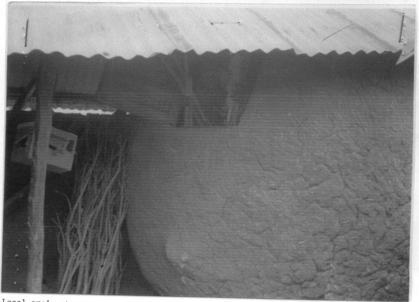
Local grain storage structure at Ndalohe in Niger State
