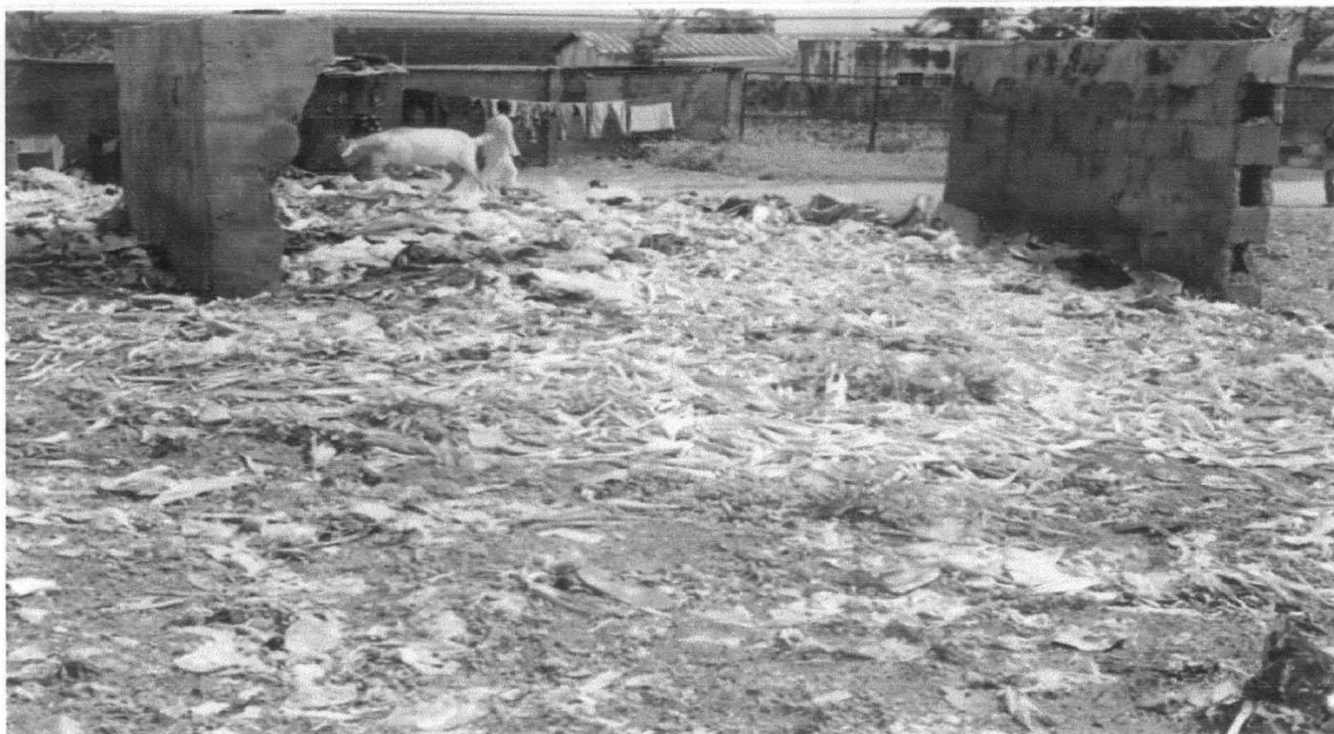
Plate IV: Unmaintained Public Refuse Facility in Bida
