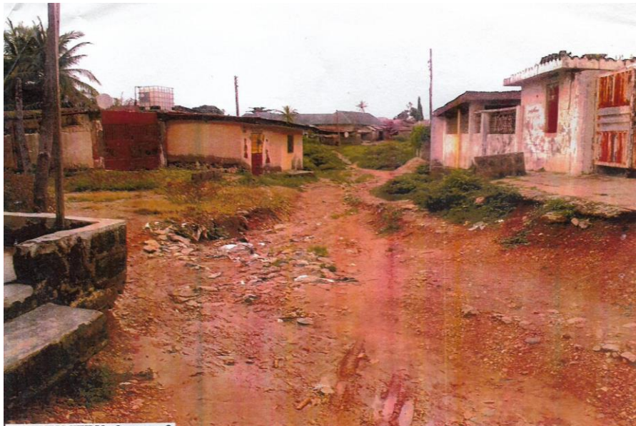
Plate II: The condition of road in the area
