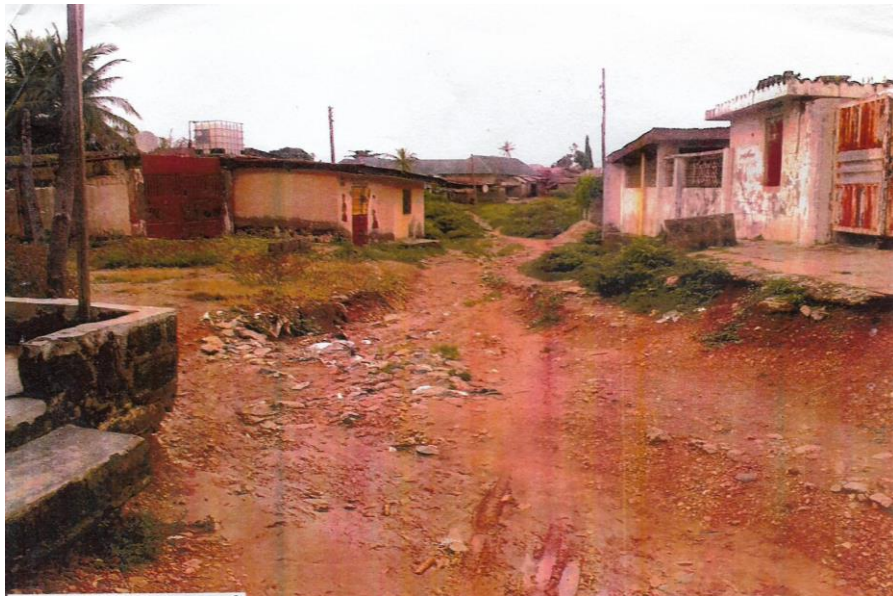
Plate II: The condition of road in the area
