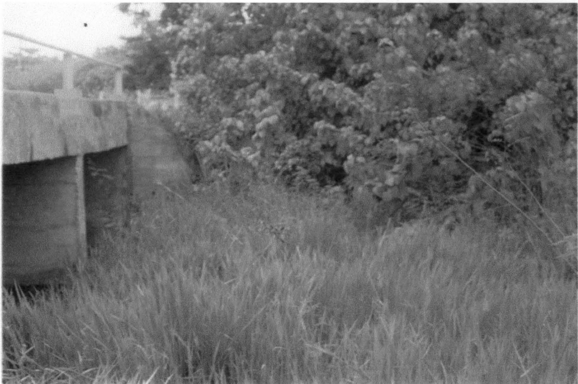
Plate 7:- Another Source of Water into the Dam
