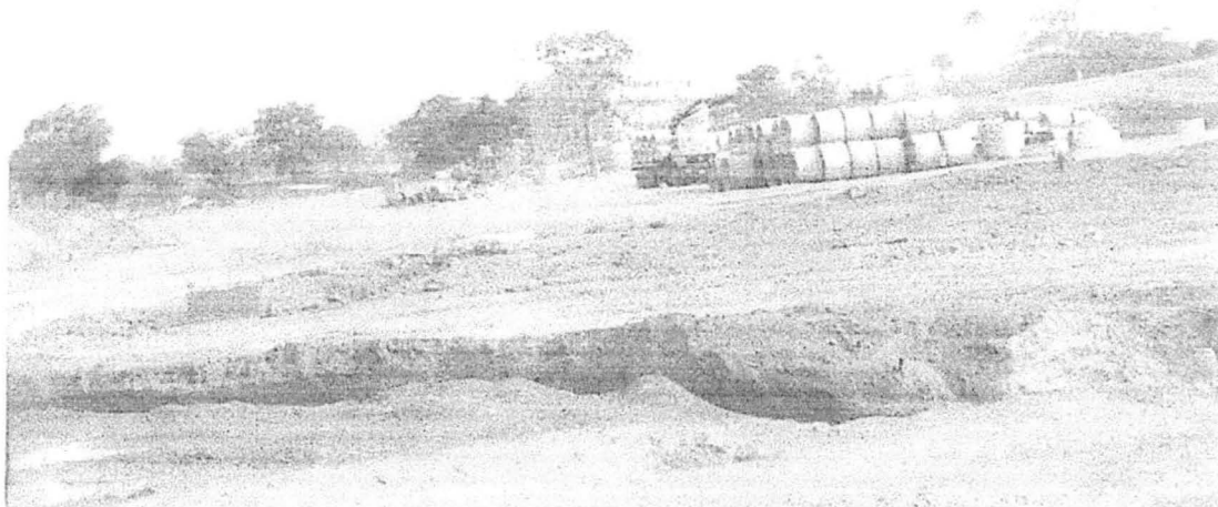
Plate 4.2 De-vegetation area in Gwarinpa District in quest for provision of infrastructures.
