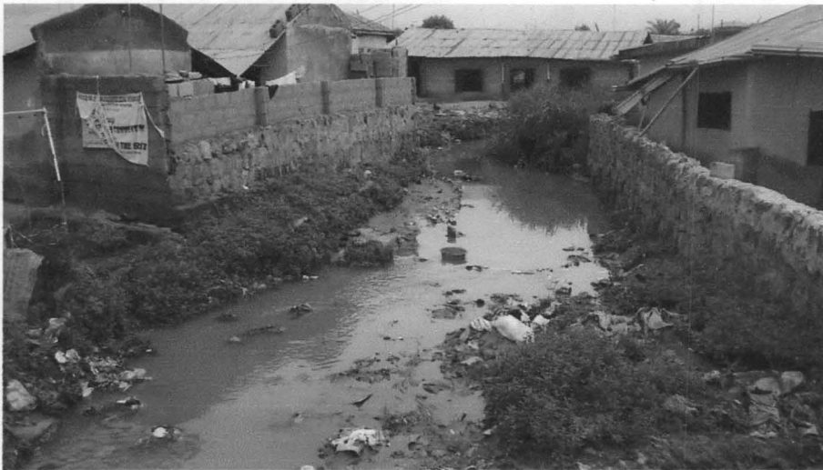
Plate XIV: Un-channelled open drain
