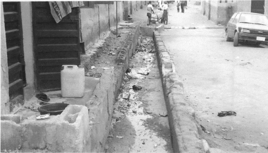
Plate XIII: Channelled but open drain
