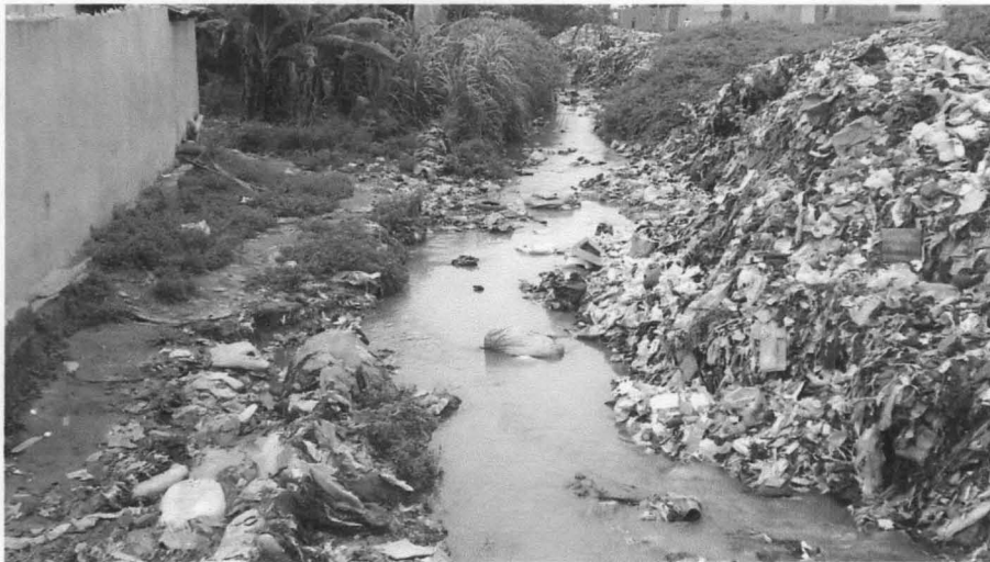
Plate XII: Picture showing Poor drainage
