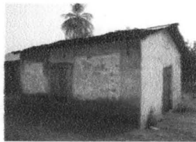
Plate 4.7.7 Primary Health center at Koriko Village
