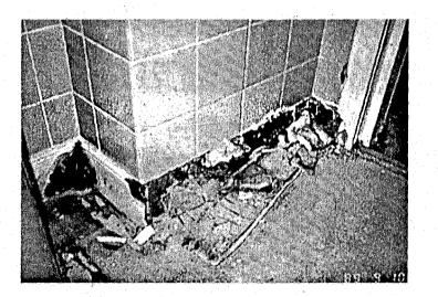
Plate 3.2 Rotting of timber skirting caused by rising damp
