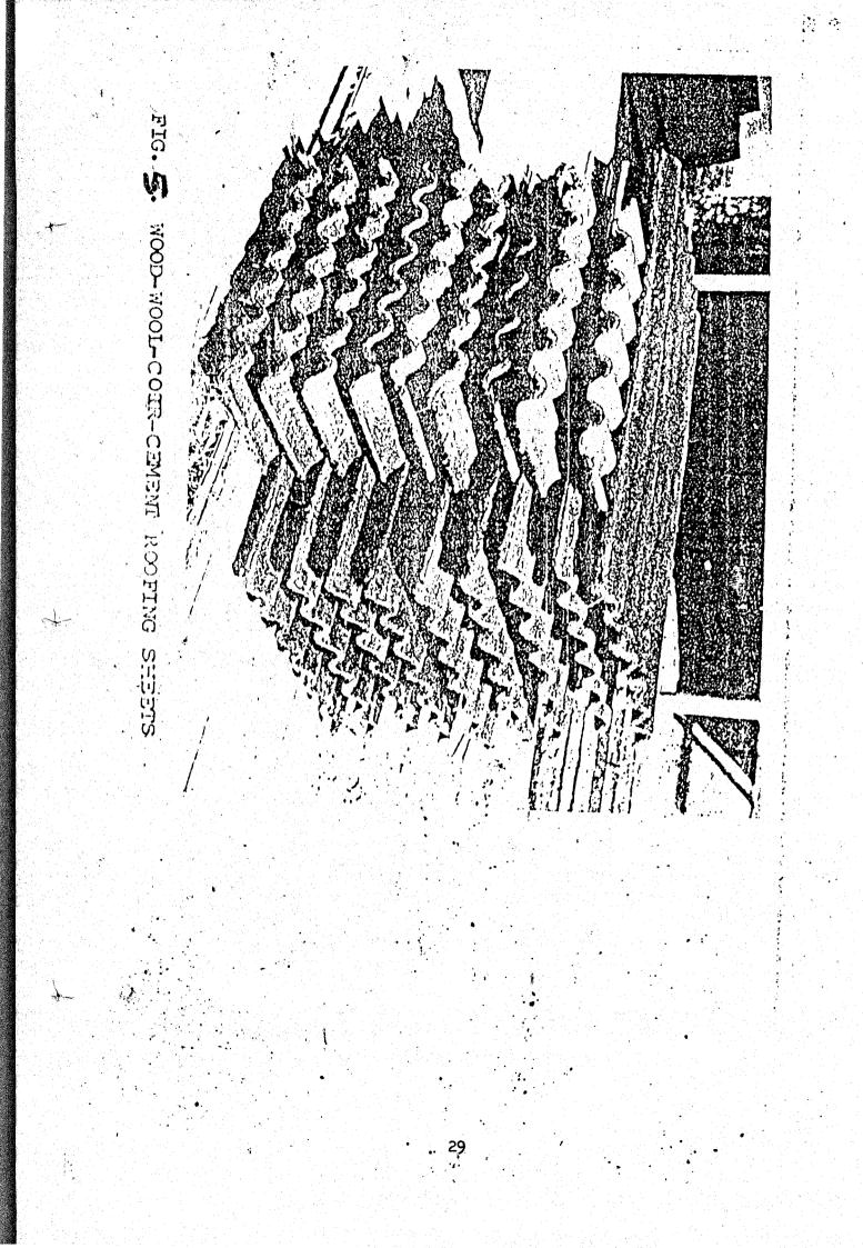
C.B.R.I has developed a building board from fibre and cement. This flat board could be used as until panels for timber or RCC or metal frame structures, as permanent stuttering for concrete, erection of free standing and sound proof partitions for false ceilings as well as roofs see fig 5.
