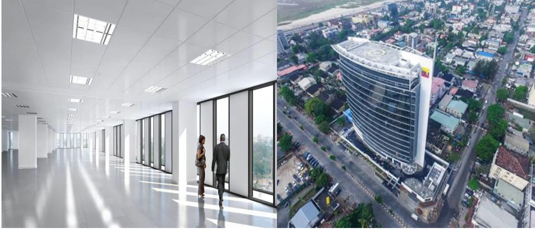
Plate V: Building Interior and Exterior Building Envelope Source: Nestoil Tower (2019)
