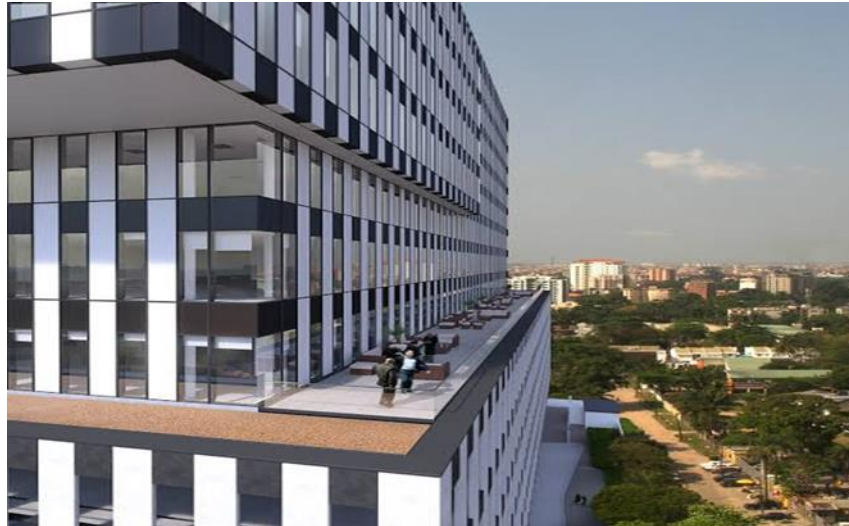
Plate IV: Curtain Walls and Balconies Source: Heritage Place (2019)
