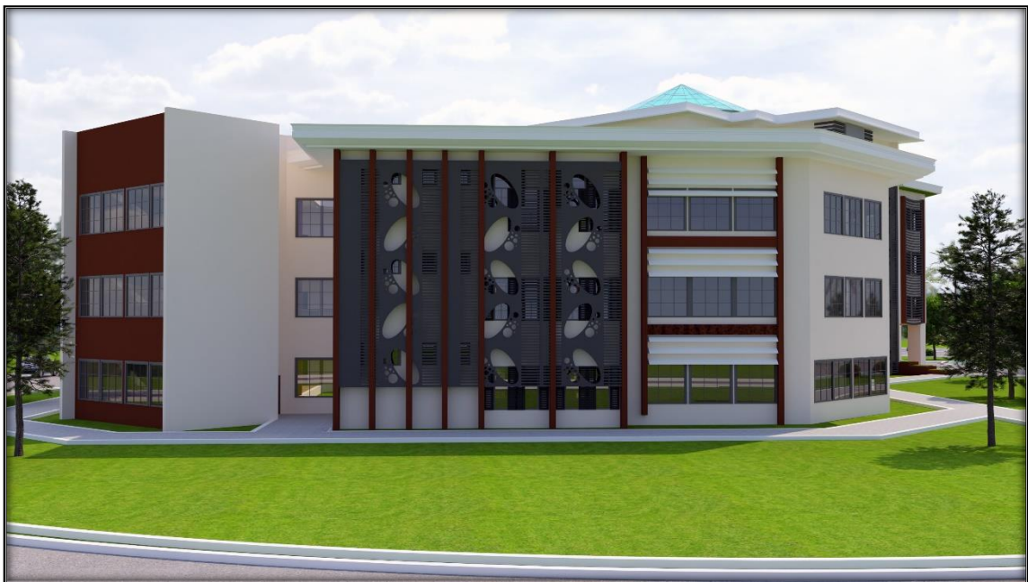
Plate VII: The use of vertical and horizontal shading devices, as well as an aluminium panel shading from sun and dust (Source: Author, 2019)
