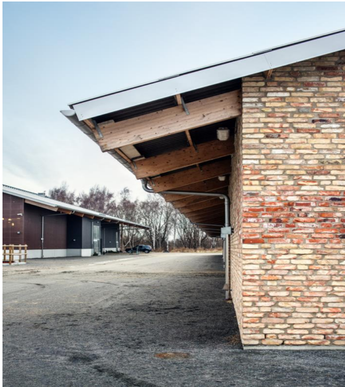
Plate VIII: A view of the barn showing local building materials (Source: Nathan, 2015)
