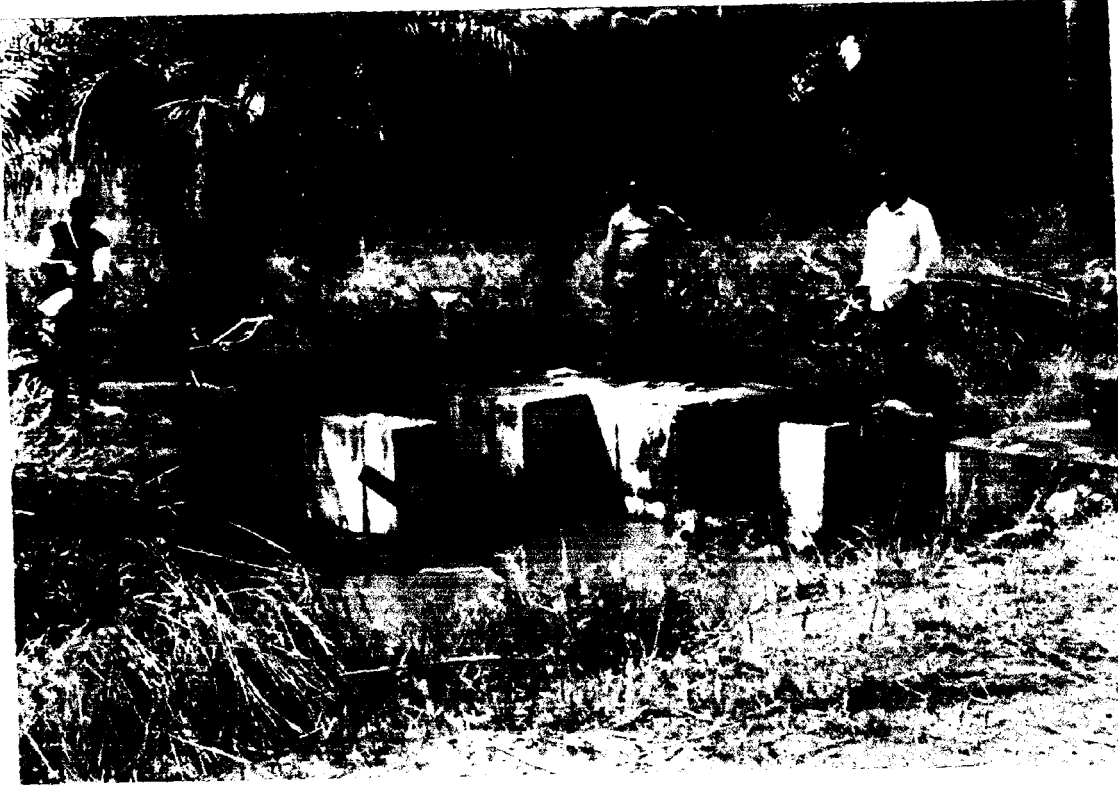
Diversion structure with washed away channel embankment
